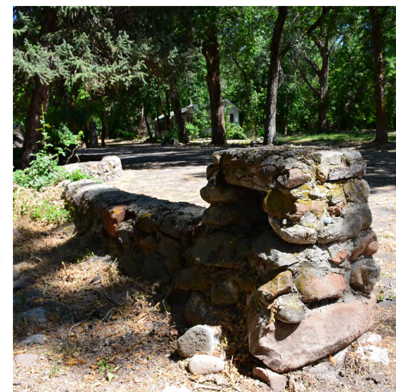
Stone wall on site
