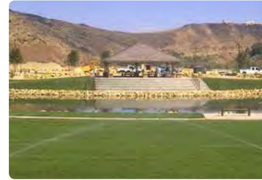
Local Project Success: Washington Fields Detention Basin, Washington Utah Photography by URS
