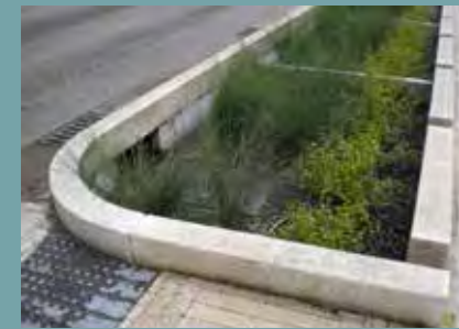
A rain garden works by capturing stormwater to irrigate plants, while at the same time reducing runoff and filtering the water.
