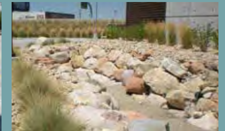
Landscaping can creatively incorporate detention basins to reduce runoff and filter stormwater.
