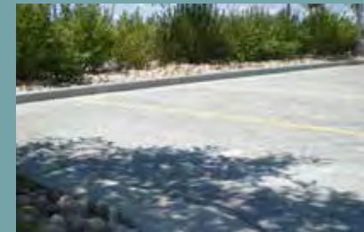
Pervious pavement is an effective way to reduce runoff where hard surfaces are needed. Pervious pavement does require periodic maintenance to preserve its porosity and effectiveness.
