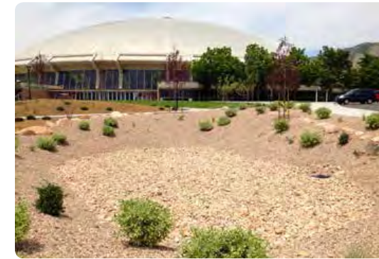
Local Project Success: Huntsman Center Stormwater Detention Basins University of Utah Photography courtesy of the University of Utah
