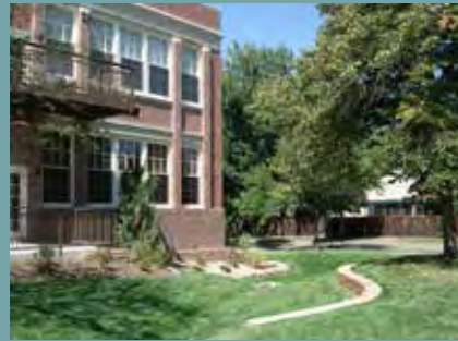
This site incorporates a natural stormwater detention basin into the landscaping.
